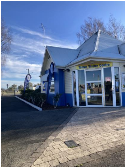
Visitor Centre access no steps
